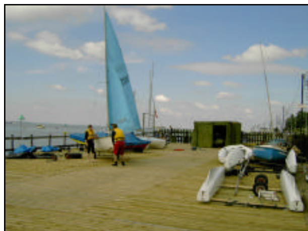
Jetty: New Decking
